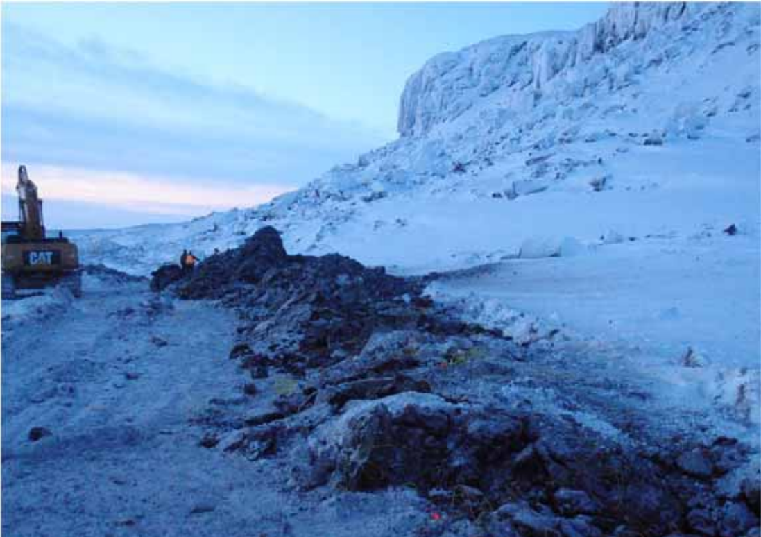
Photo 11: ~ WNW view of the Doris North Diversion Berm after early afternoon blasting. Note the large quantity of frozen overburden encountered along this section (near the east to east central portion of the alignment).
