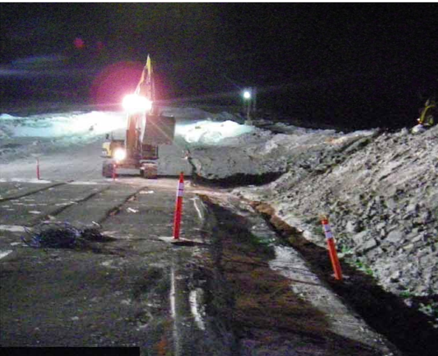
Photo 16: Downstream side of key trench with snow cleared in preparation for transition material placement.
