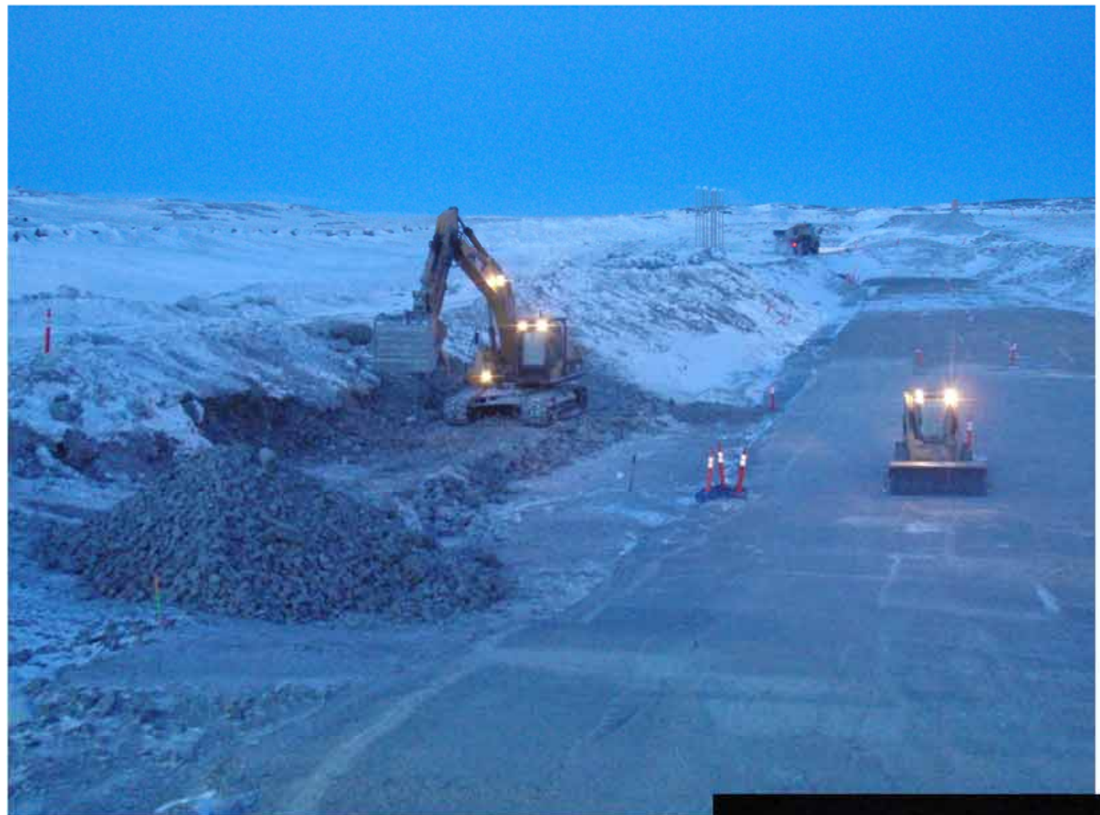
Photo 14: ~NE view of the 325 excavator placing transition material around station 1+00.
