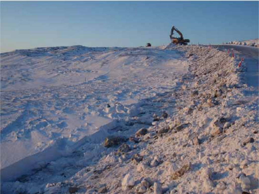
Photo 1: ~ WNW view of the 325 excavator working on snow clearing activities along the side slopes of the Secondary Road, taken in the am.
