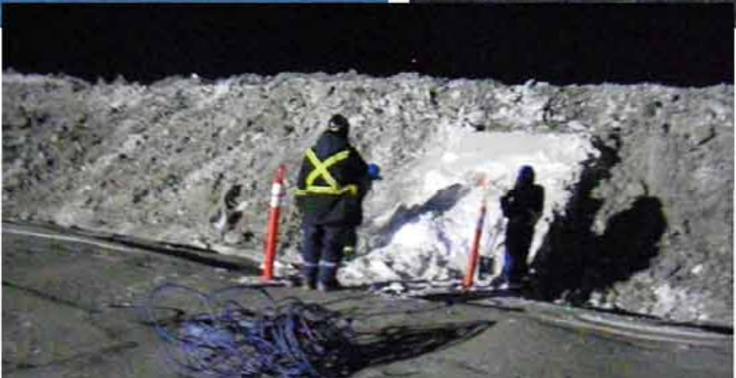
Photo 15: Labourers cleaning snow away from the thermistor cables at station 1+30.
